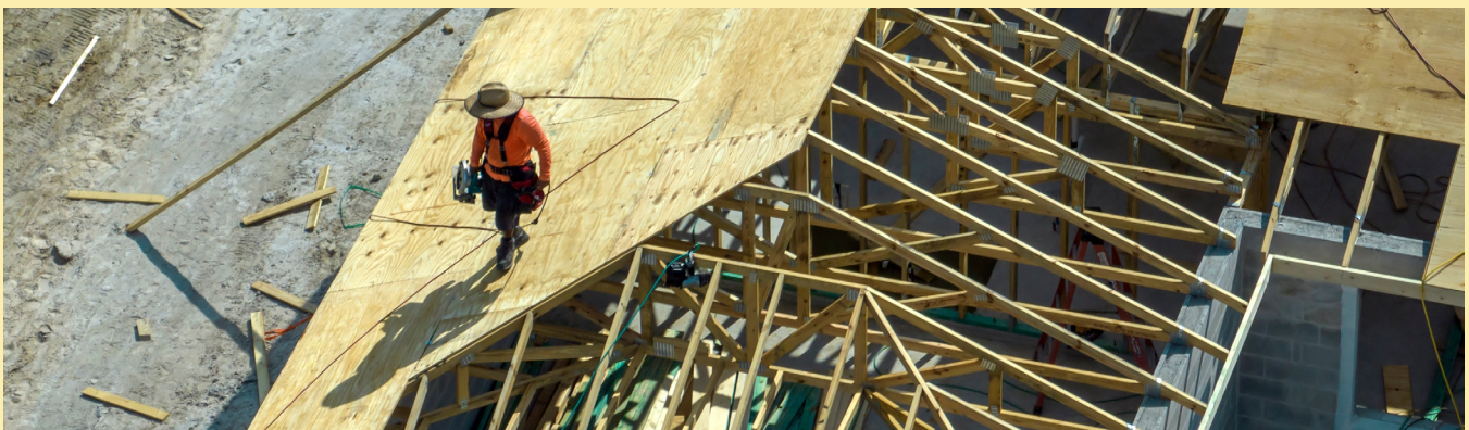
Construction worker in Sarasota, Florida, U.S. Photo by Bilanol .
